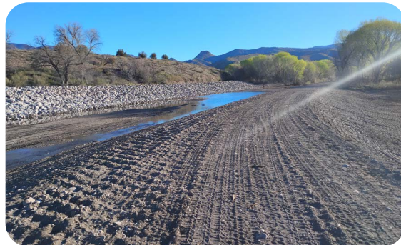
Bank Stabilization. Photo by Gregor Hamilton
